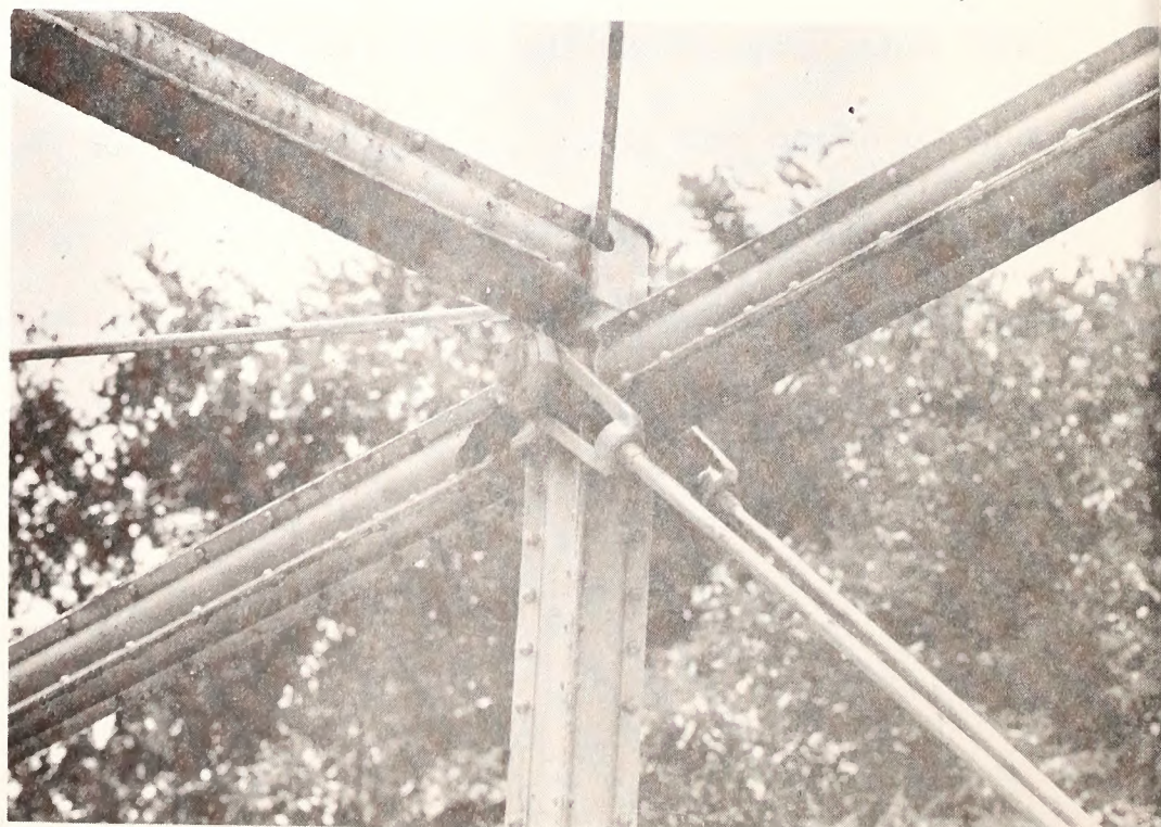
Right, a detail of a cast iron joint in the 1891 bridge.
